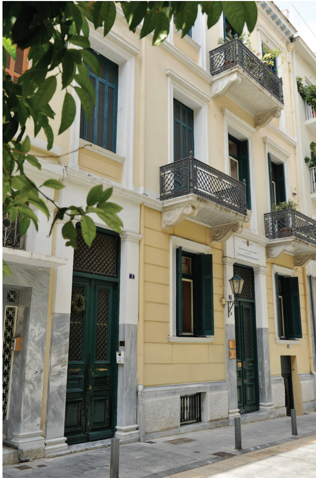
Fig. 10. The HFRC's building in Plaka, central Athens.
