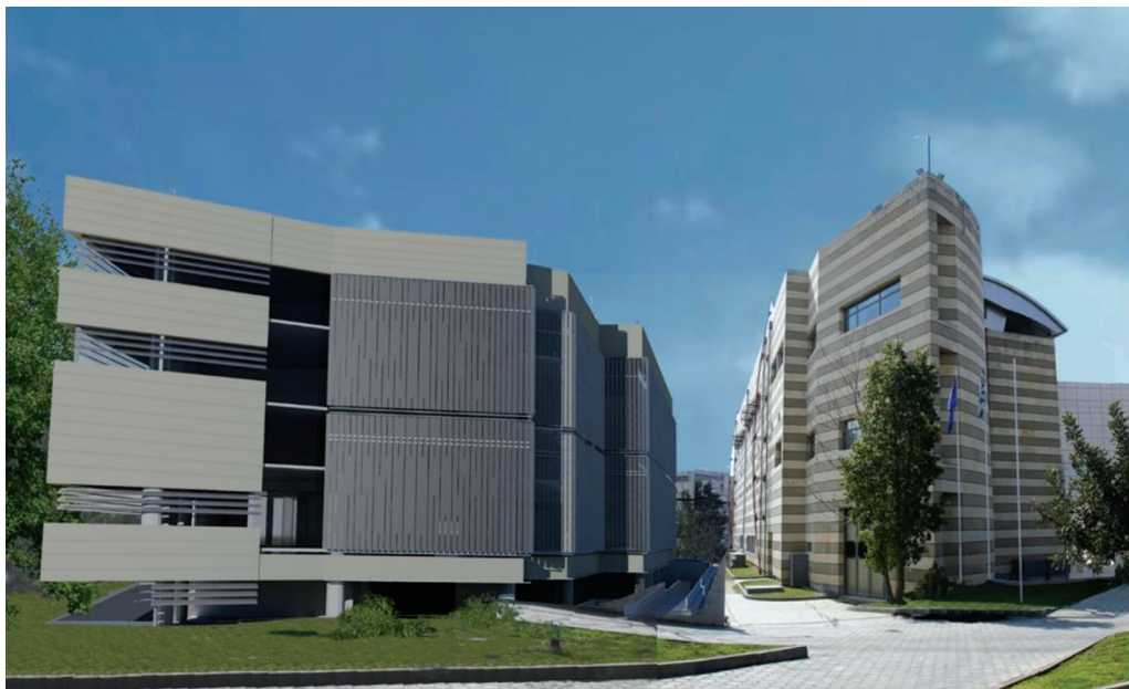
Fig. 9. General view of the existing (right) and the planned new facilities of BRFAA (left).
